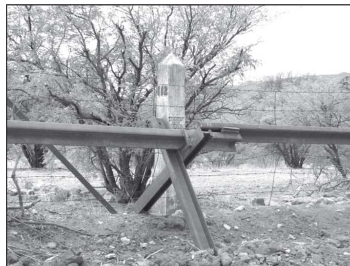
A recently fortified portion of the border west of Lochiel, Arizona, has altered the character of International Boundary Monument No. 112, erected during the 1890s expedition that attempted to relieve some of the disarray that had surfaced since the original 1850s boundary survey.
