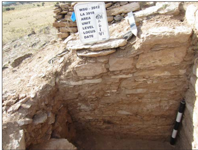
External wall face of the Largo Gap great house, displaying Chacoan-style Type II masonry, based on Lekson's (1986) masonry classification scheme; view to the south. (Photograph by Patrick Dolan.)
